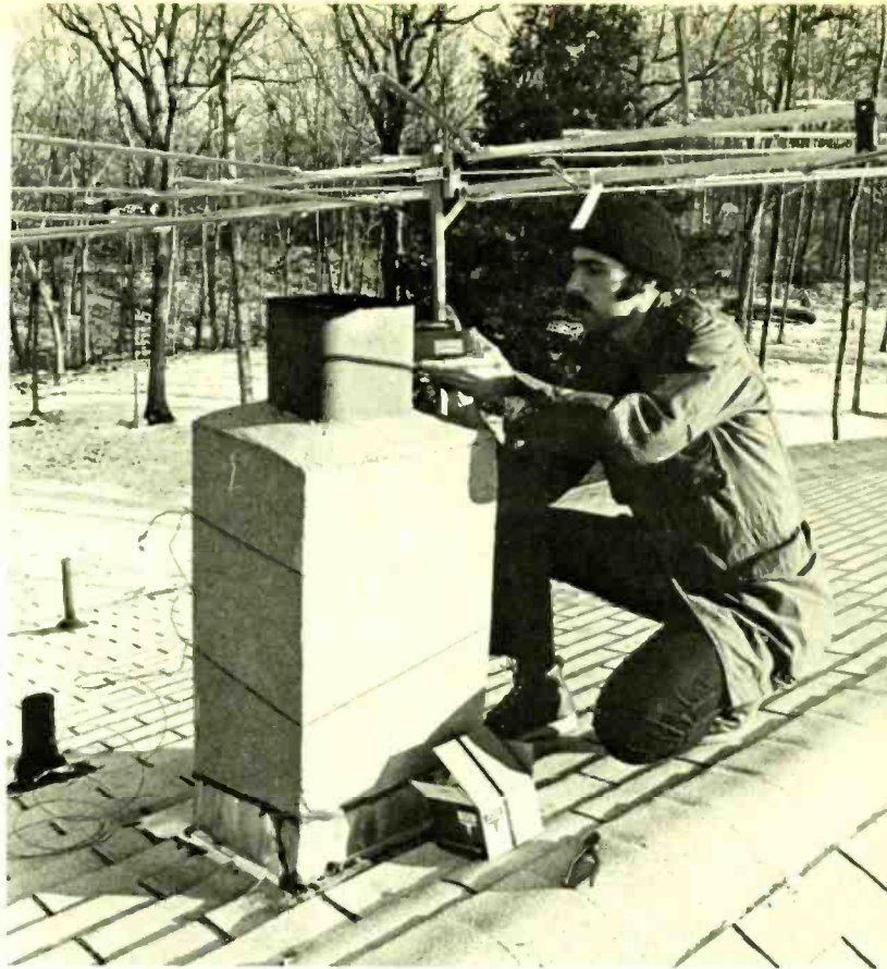
BOOSTER MOUNTS ON MAST and connects between lead in and transmission coax. In typical installations the antenna should be mounted further above the chimney.
